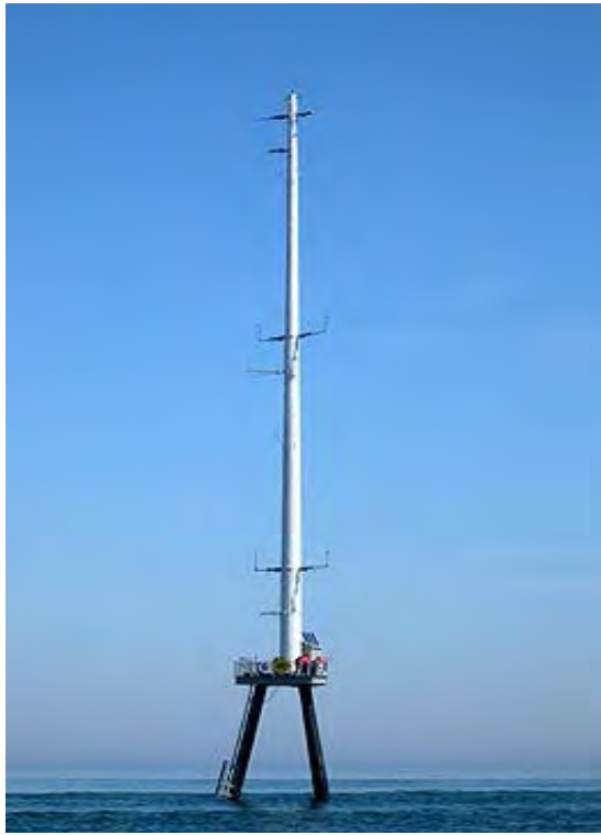
Figure 3-5 Example of Monopole-mast Meteorological Tower
